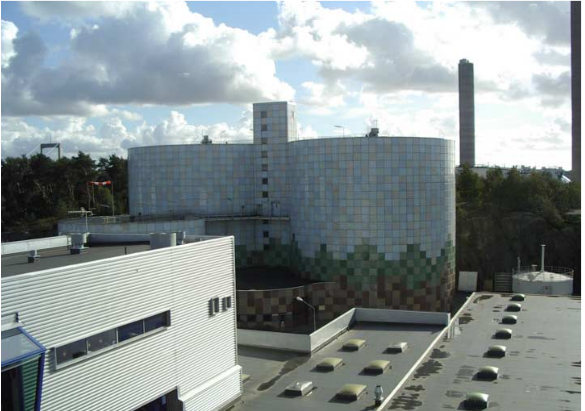
Gothenburg's biogas digesters...
